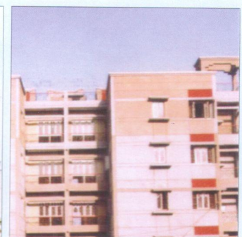
Gurgaon, Ph-I : 1088 DUs Completion Year : July, 1999
