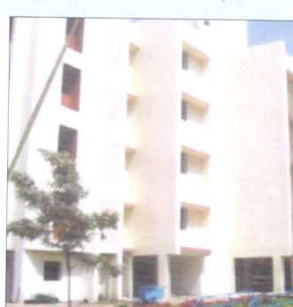
Pune, Ph-II : 148 DUs Completion Year : December, 2008
