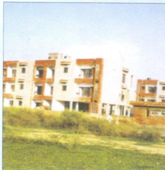
Chandigarh : 305 DUs Completion Year : May, 2000
