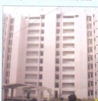
Mohali, Ph-I : 603 DUs Completion Year : April, 2013
