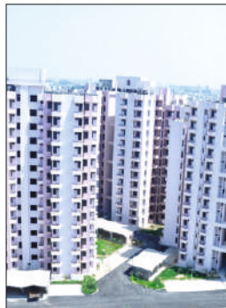
Mohali Ph-II : 615 Dus Completion Year : 2017
