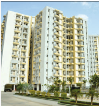
Jaipur, Ph-II : 572 DUs Completion Year : March, 2012
