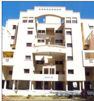
Hyderabad, Ph-II : 380 DUs Completion Year : October, 2012
