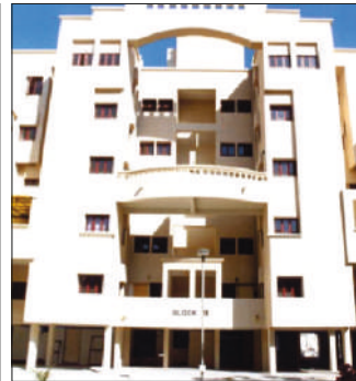
Hyderabad, Ph-I : 344 DUs Completion Year : July, 2001
