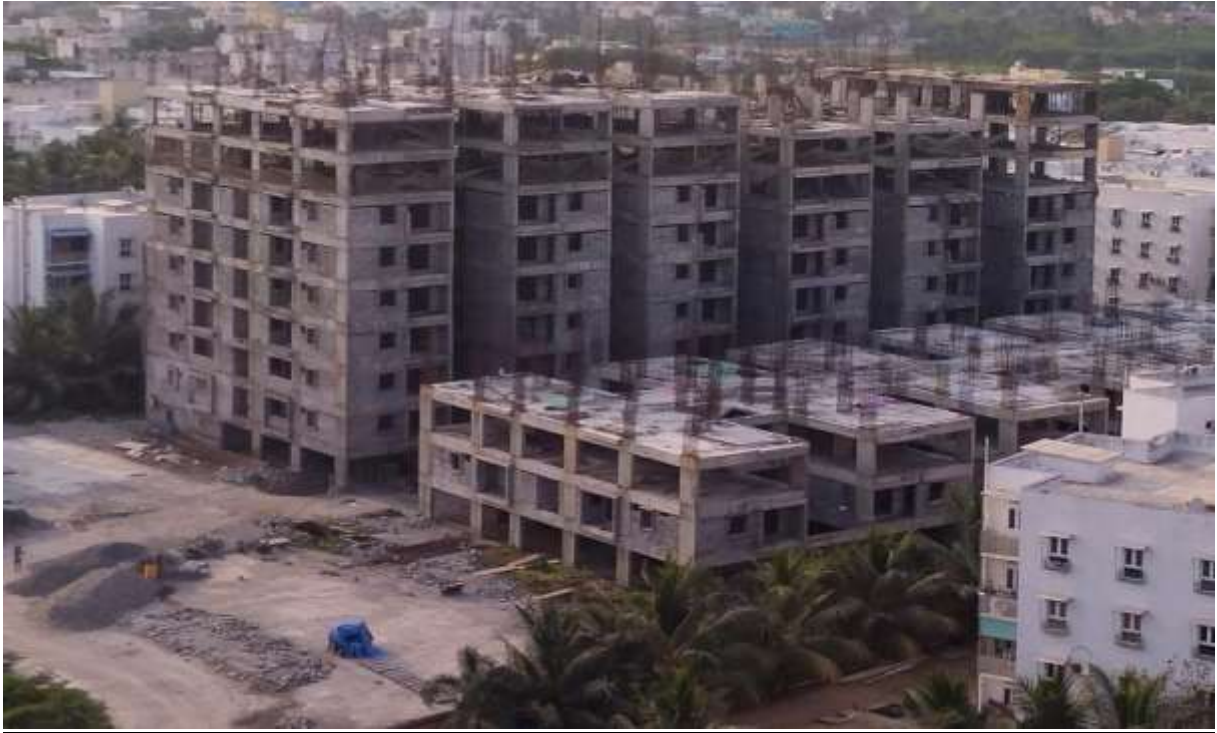
View of B1 Block & B2 Block
