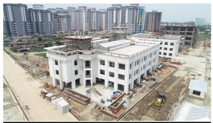
COUMNITY 3<sup>RD</sup> FLOOR ROOF SLAB SHUTTERING & EINFORCEMENTWORK INPROGRESS.
