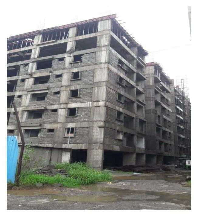
Community Hall: Columns upto Fourth floor level 100% completed. Shuttering and Barbending works for Fourth floor level slab 85% completed and balance work on progress.
