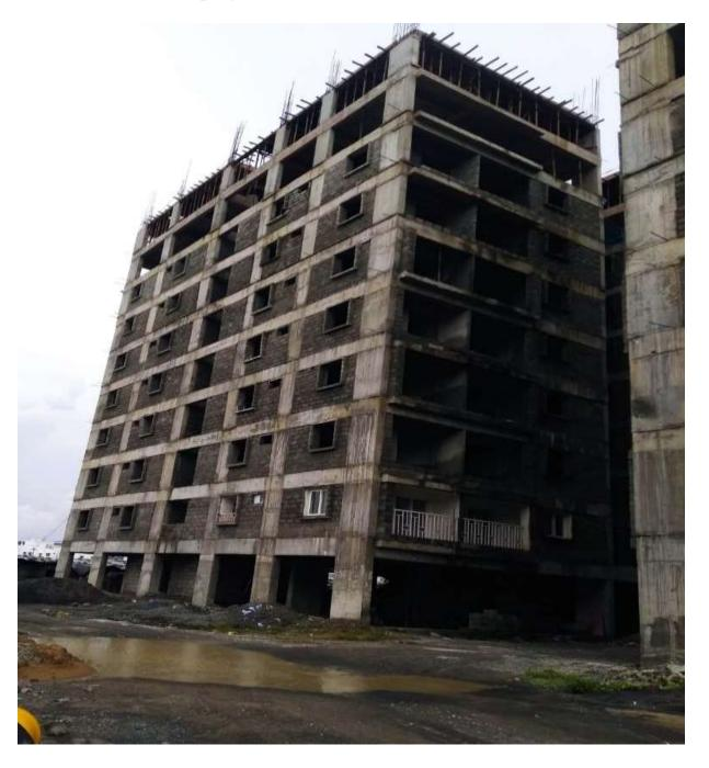
Block C2: Ninth floor level slab First Half Concrete casting 100% completed. Shuttering & Barbending works for 2<sup>nd</sup> Half of Ninth floor level slab 80% completed and balance work on progress. Columns upto Tenth Floor level 100% completed.
