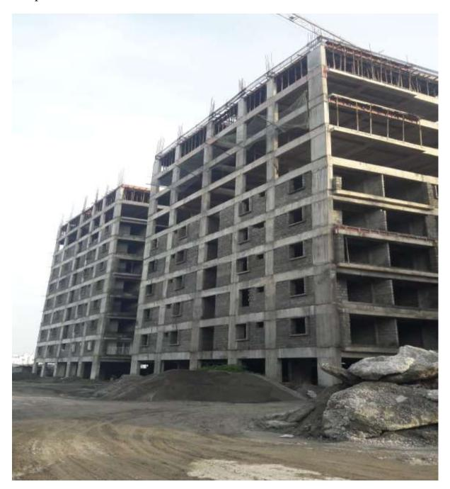
Block C3: Columns upto Seventh Floor level 100% completed. Shuttering & Barbending works for 1<sup>st</sup> Half of Seventh floor level slab 10% completed and balance work on progress.
