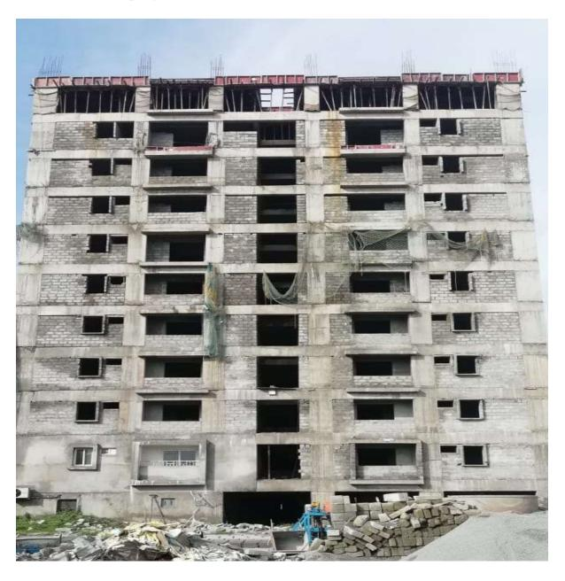
Block B2: Third Floor Level slab concrete casting 100% completed. Bar bending works for Columns up to fourth floor level on progress.
