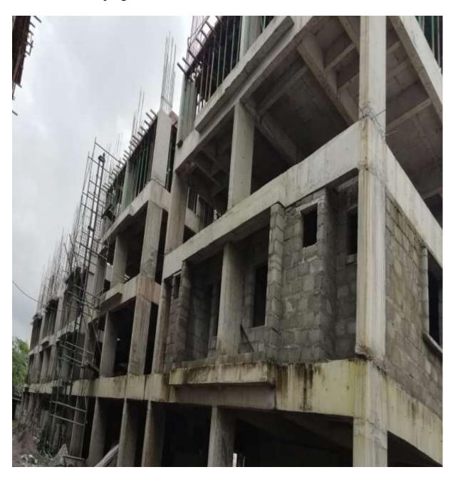
Block B1: Columns upto Terrace Floor 75% completed. Shuttering and Barbending works for 1<sup>st</sup> Half of Terrace floor level slab 80% completed and balance work on progress.
