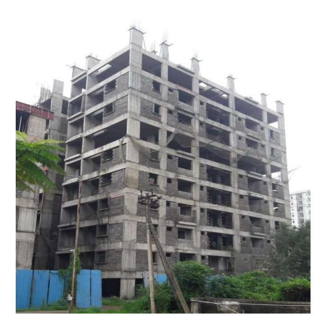
Block D3: Eight Floor Level slab  $1^{st}$  half concrete casting 100% completed. Shuttering & Barbending works for  $2^{nd}$  half of Eight floor level slab 85% completed and balance work on progress.
