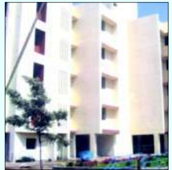
Pune, Ph-II : 148 DUs Completion Year : December, 2008
