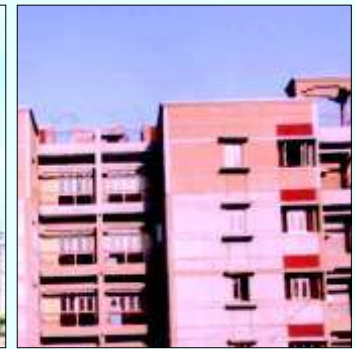
Gurgaon, Ph-I : 1088 DUs Completion Year : July, 1999
