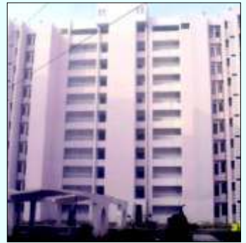
Mohali, Ph-I : 630 DUs Completion Year : April, 2013
