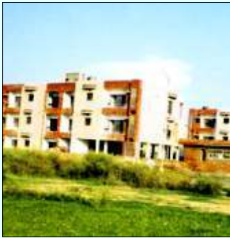
Chandigarh : 305 DUs Completion Year : May, 2000
