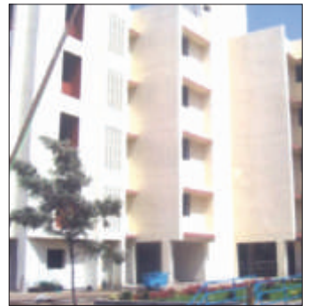
Pune, Ph-II : 148 DUs Completion Year : December, 2008
