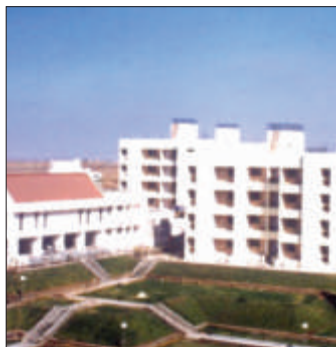
Pune, Ph-I : 159 DUs Completion Year : January, 2003
