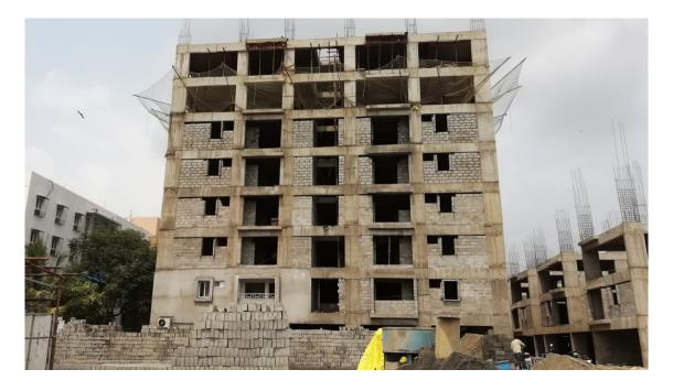
Block B2: Third Floor Level slab concrete 100% completed. Bar bending works for Columns up to fourth floor level on progress.
