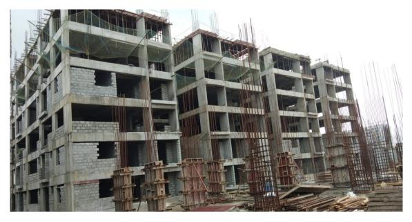
Block D3: Fourth Floor Level slab concrete casting 100% completed. Shuttering works & Barbending works for 1<sup>st</sup> Half of Fifth floor level slab 10% completed..
