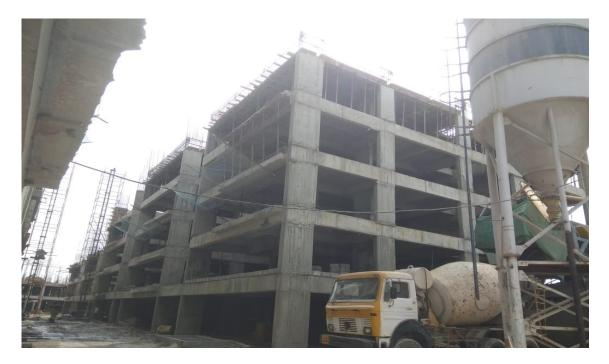
Block D1: First Floor Level slab concrete casting 100% completed. Shuttering works & Barbending works for 1<sup>st</sup> Half of Second floor level 15% completed..
