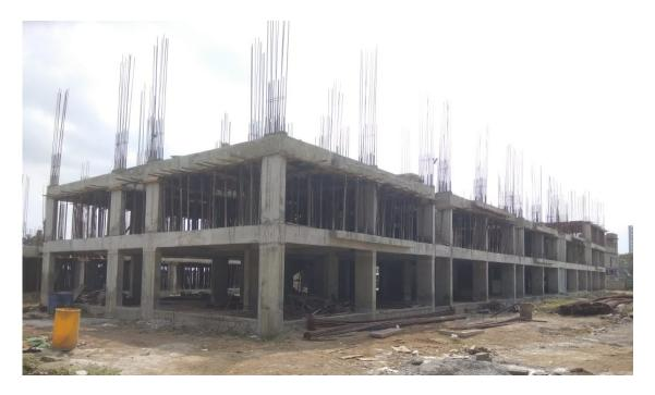
Block A2: First Floor level slab concrete casting 100% completed. Shuttering and barbending work on progress for 1<sup>st</sup> Half of Second Floor level.
