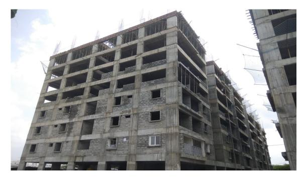
Block C2: Sixth Floor level slab  $1^{st}$  Half concrete casting completed &  $2^{nd}$  Half concrete casting 50% completed. Shuttering and Barbending work on progress for  $1^{st}$  half of Seventh Floor level slab.
