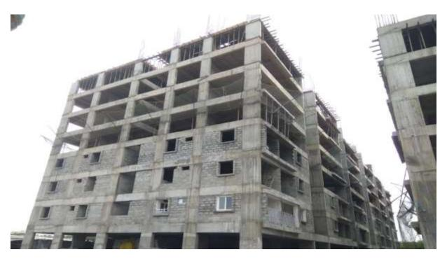
Block C2: Sixth Floor level slab First half concrete 100% completed. Shuttering and Barbending work on progress for Second half of Sixth Floor level slab.
