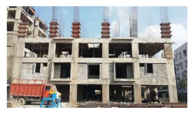
Block C1: Columns up to eight floor level 50% completed and balance work on progress. Shuttering work on progress for First half of Eight Floor level slab.
