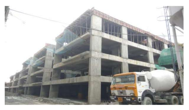
Block D1: First Floor Level slab 1<sup>st</sup> Half concrete completed and for 2<sup>nd</sup> half Shuttering works & Barbending works 90% completed..
