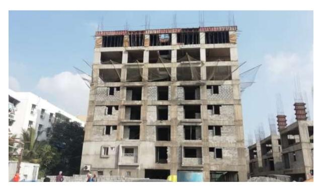
Block B2: Third Floor Level slab concrete 100% completed. Shuttering and Bar bending works for Columns up to fourth floor level on progress.
