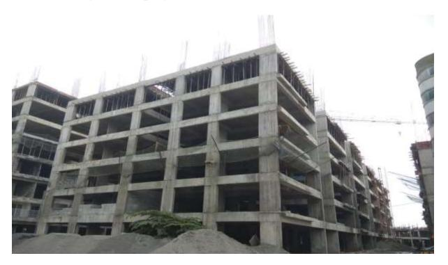
Block C3: Third Floor Level slab concrete 100% completed. Fourth Floor Level slab First Half concrete completed .
