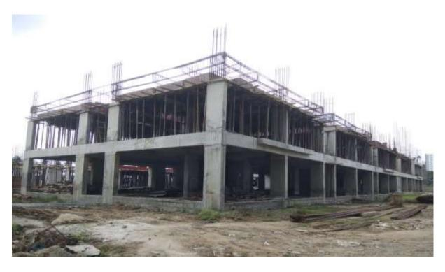
Block A2: First Floor level slab concrete 1<sup>st</sup> Half completed & in 2<sup>nd</sup> half beam shuttering and barbending fabrication works on progress.
