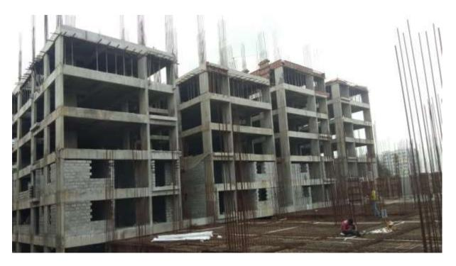
Block D3: Fourth Floor Level slab 1<sup>st</sup> Half concrete completed and for 2<sup>nd</sup> half Shuttering and bar bending work 95% completed.
