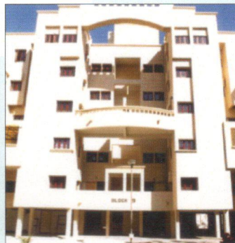
Hyderabad, Ph-I : 344 DUs Completion Year : July, 2001
