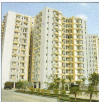
Jaipur, Ph-II : 572 DUs Completion Year : March, 2012
