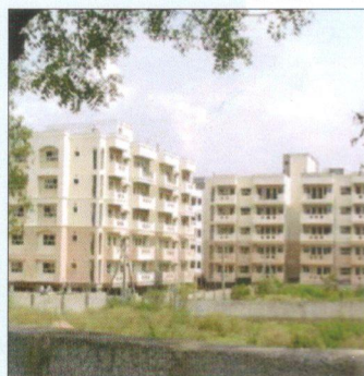
Hyderabad, Ph-II : 380 DUs Completion Year : October, 2012
