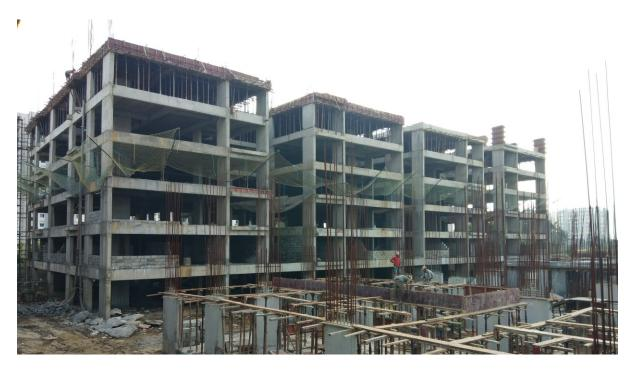
Block D3: Fourth Floor Level slab 1<sup>st</sup> Half concrete completed and for 2<sup>nd</sup> half columns concrete work 90% completed.
