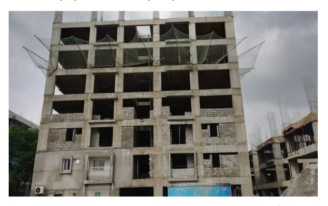
Block B2: Third Floor Level slab concrete 1<sup>st</sup> Half completed & in 2<sup>nd</sup> half floor Shuttering & Barbending works 80% completed.
