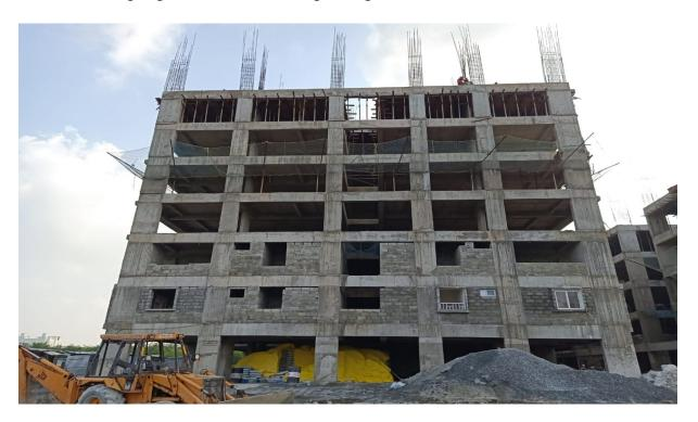
Block C2: Fifth Floor level slab 1<sup>st</sup> Half concrete completed and in 2<sup>nd</sup> Half shuttering & barbending works 85% completed.
