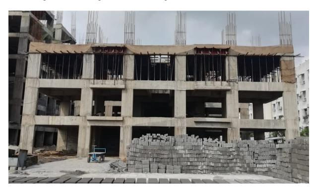
Block C1: Seventh Floor level slab 1<sup>st</sup> half concrete completed. Barbending works are on progress for columns upto Eight floor.
