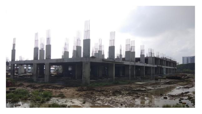
Block A2: First Floor level slab concrete 1<sup>st</sup> Half completed & in 2<sup>nd</sup> half beam bottom shuttering work on progress.
