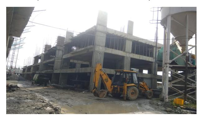
Block D1: First Floor Level slab 1<sup>st</sup> Half concrete completed and for 2<sup>nd</sup> half barbending works are on progress
