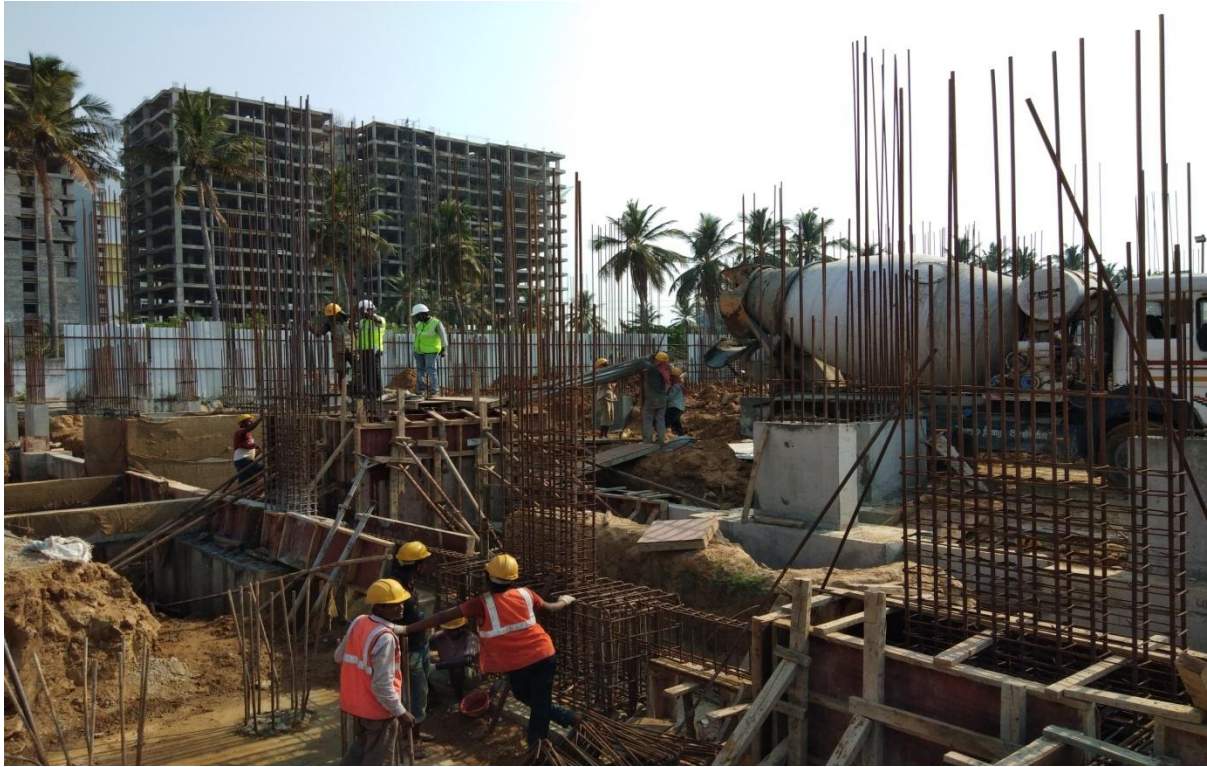
In Block D2 Pile Cap Works are in progress.
