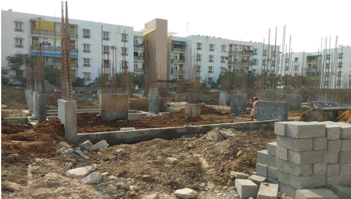
In Block B2 Piling Work in progress.
