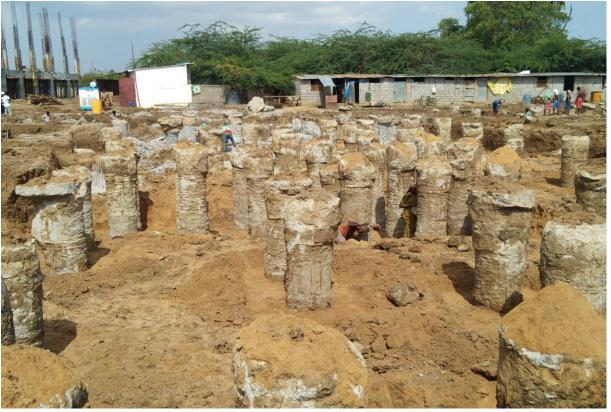
In Block A2 Excavation works, PCC Work, Pile chipping work in progress.
