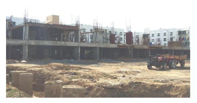
In Block B2 Excavation Work for Pile Cap Works on process.
