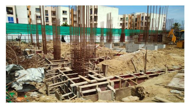
In Block B1 shuttering work for First floor level slab is on progress.
