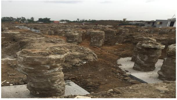
In Community Centre Pile cap Concrete casting works , pile chipping work up to cut off level & Shuttering work and bar bending works for pile caps on progress.
