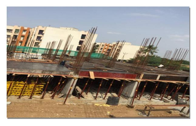
In Block D3 Pile Cap Concrete Work, Column Concrete upto Stilt floor & Backfilling on Progress for Second half of the Block
