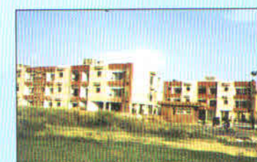
CHANDIGARH - 305 DUs Completion Year : 2000
