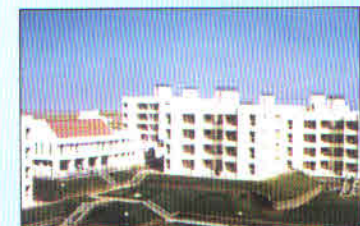
PUNE (Ph-I) - 159 DUs Completion Year : 2003
