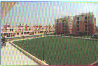
LUCKNOW - 130 DUs Completion Year : 2008
