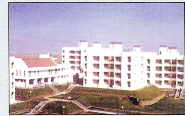
PUNE (Ph-I) - 159 DUs Completion Year : 2003
