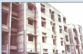
GURGAON (Ph-II) - 852 DUs Completion Year : 2002
