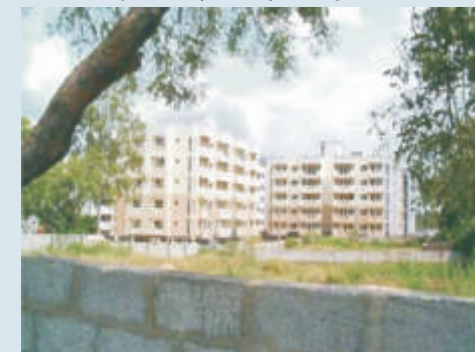
Hyderabad (Phase-II) Housing Scheme : 178 Flats
