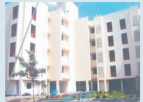
Pune (Ph-II) Housing Scheme : 148 Flats
