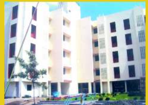
Pune (Ph-II) Housing Scheme : 148 Flats
